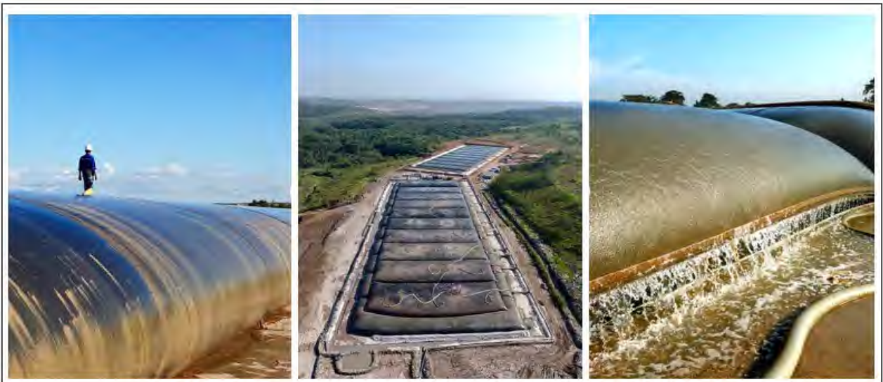
Figure 19: TenCate Geotube used for dewatering (Reference: TenCate Geosynthetics)
